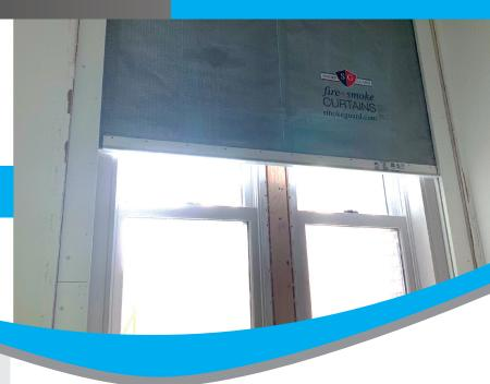
Applications. The M1000 fulfills a niche ignored by most other products. As an alternative means of providing a fire-rated passive system, the M1000 may be used; in conjunction with fire control systems, on its own to protect areas where a fusible link release system is appropriate, or at exterior windows as protection against radiant heat.
