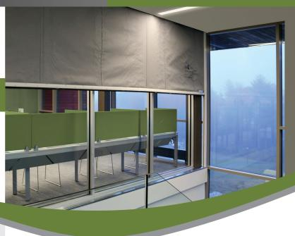
Codes and Standards. M2500 fulfills IBC requirements to provide an opening protective, where these assemblies are permitted as passive barriers used in conjunction with smoke control systems. This fire or smoke-rated curtain system can serve as an opening protective for counter top, openings in corridors, and applications in atriums.
