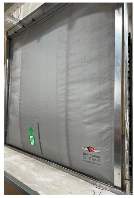
**System Operation.** The system is deployed on an alarm signal from the local smoke detector or from a fire control panel. System power requirement is 120/240-volt AC. The unit is also equipped with a 12-volt DC battery back-up system that is maintained by the electronic controls. When required, the system can also be connected to building standby power. The controls include a universal power supply that can be adapted to foreign electrical current requirements.
